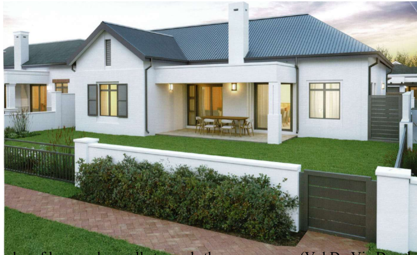
Examples of low garden walls towards the open spaces (Val De Vie Development)
