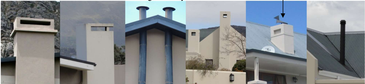
Figure 12 Examples of chimneys
